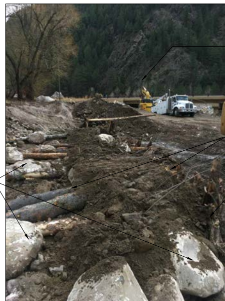
LARGE WOOD COMPLEX IN CONSTRUCTION (PHOTO SHOWS INSTALATION BIGGER THAN THOSE IN THE WALL STREET PROJECT)
