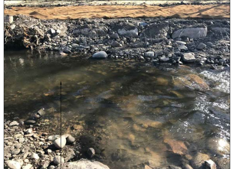
EXAMPLE 1: CONSTRUCTED POOL HEAD: RIFFLE STEEPENS AND CHANNEL CONSTRICTS AT POOL ENTRANCE
