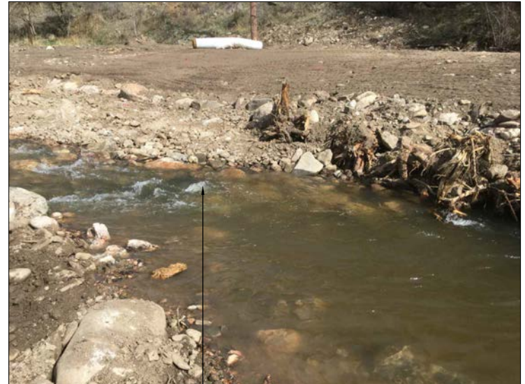
EXAMPLE 1: CONSTRUCTED POOL HEAD: RIFFLE STEEPENS AND CHANNEL CONSTRICTS AT POOL ENTRANCE
