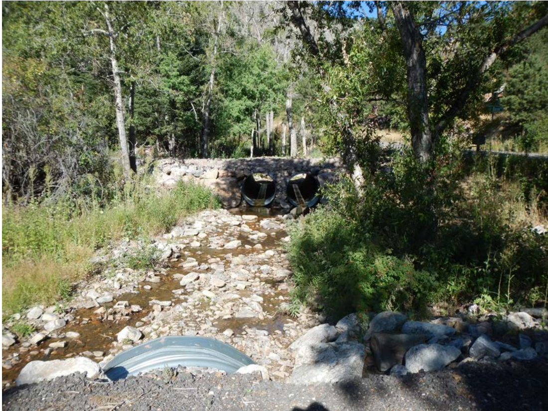
Figure 1. Coal Creek stream channel at Area 2 showing cobble boulder substrate, wide undefined channel and culverts.
