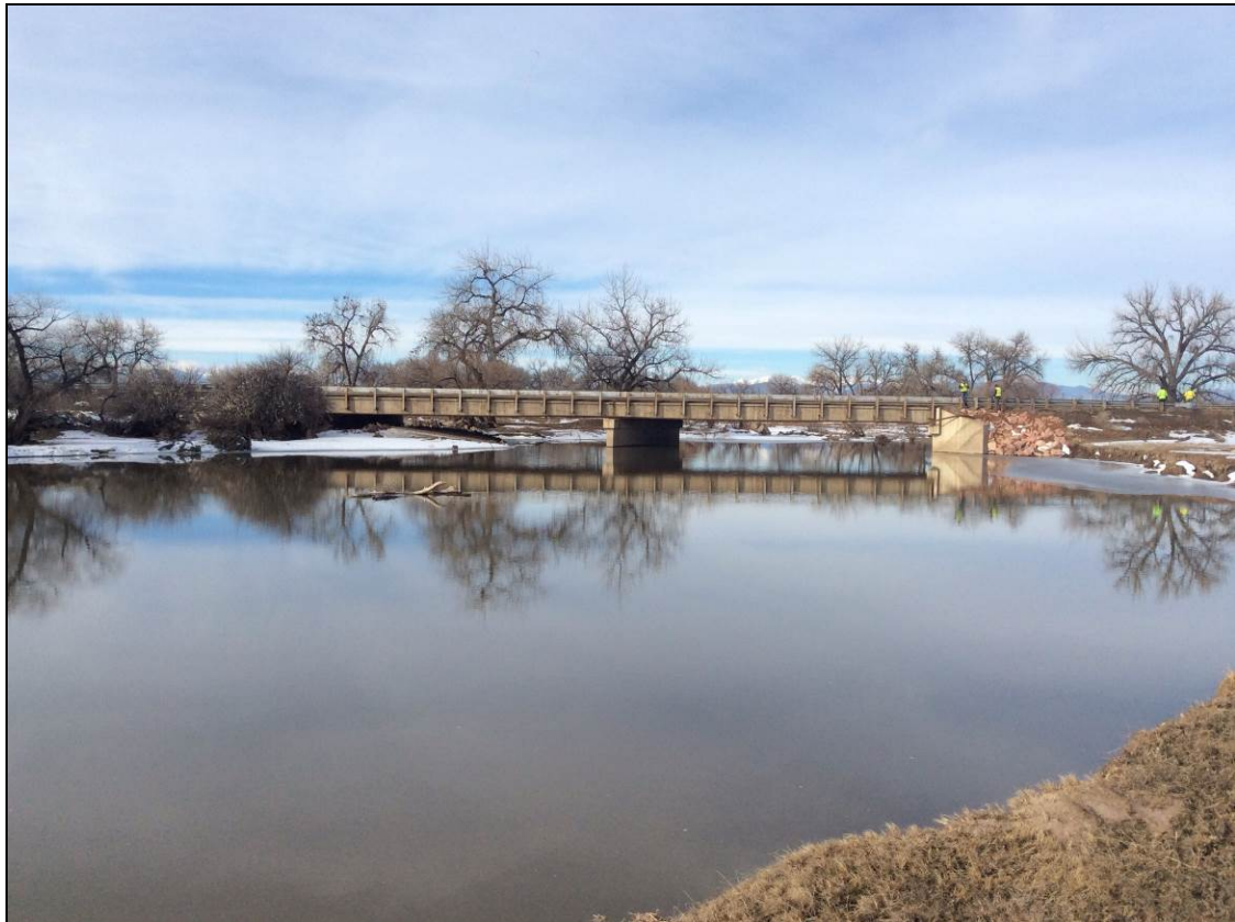
Figure 3.16. Example of post-flood stream channel at Weld County Rd 17, AHIP = 3.
