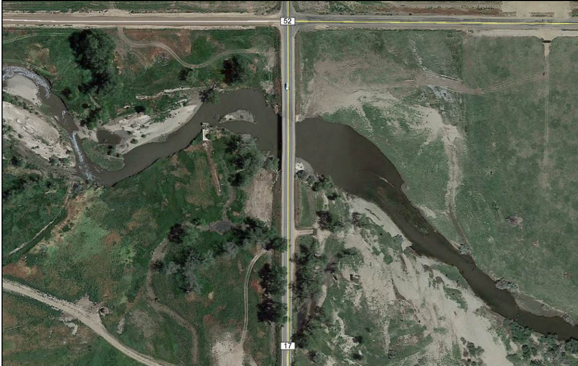
Figure 3.15. Example of post-flood stream channel at Weld County Rd 17, AHIP = 3.
