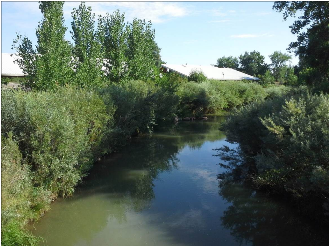
Figure 5.9. Planted riprap bank protection (left side), taken 8-29-2013, Fairgrounds Park, Loveland, CO.
