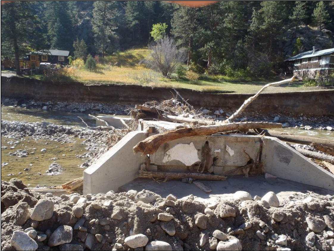
Figure 7.2. Flanked access bridge in Big Thompson Canyon.
