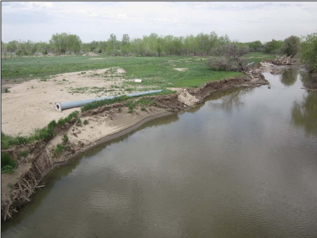
Figure 3.24. Loveland area, wide undeveloped floodplain, REIP = 4.
