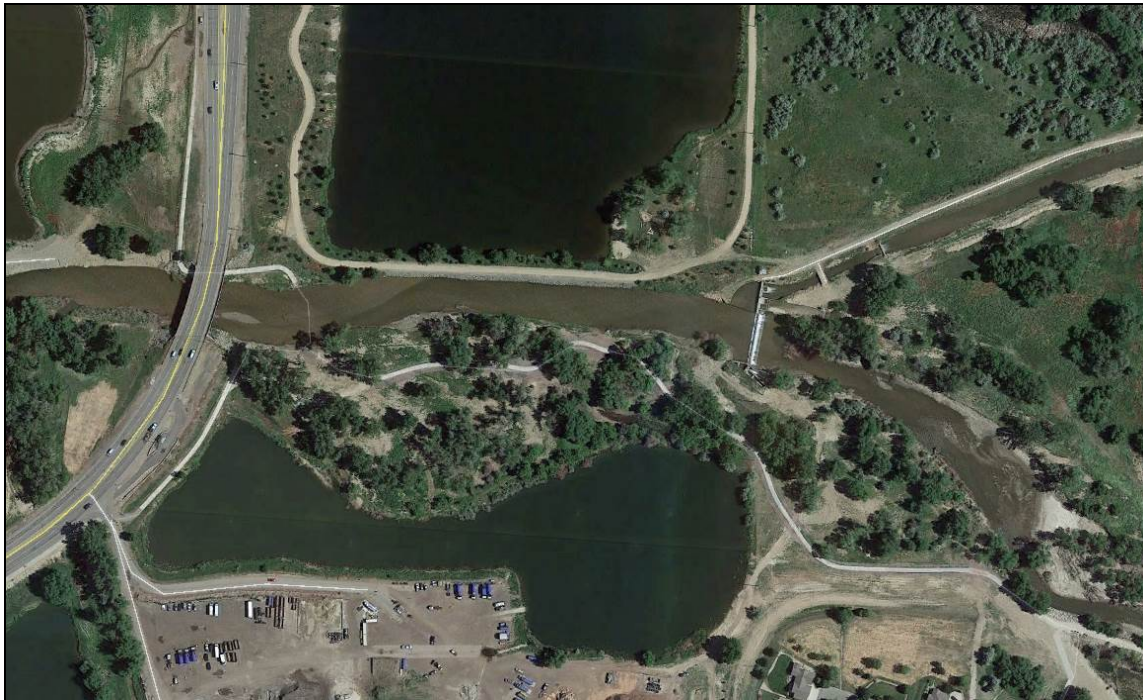
Figure 3.14. Example of post-flood stream channel at downstream of Wilson Avenue, AHIP = 1 - 3.
