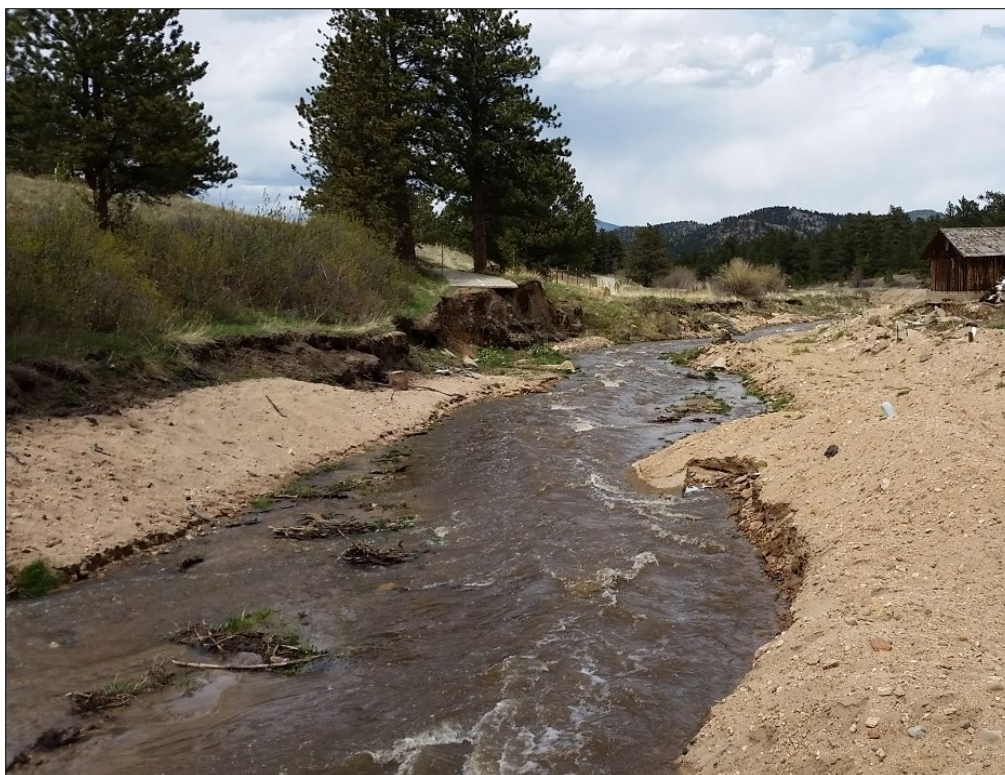
Flood Damaged Stream in Larimer County, Colorado
