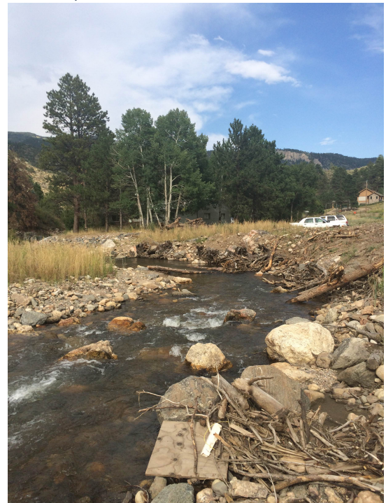
Picture 15: Engineered log jam on the North Fork of the Big Thompson River near Glen Haven, Colorado
