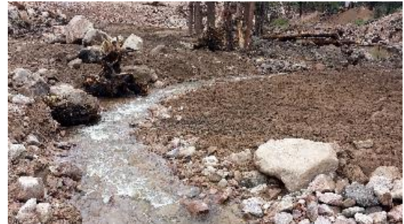
Picture 3: Constructed point bar on the Little Thompson River in Pinewood Springs, Colorado
