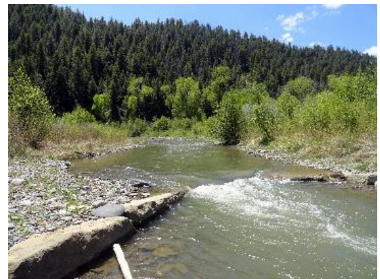
Picture 7: Cross vane on the Rio Blanco River in Pagosa Springs, Colorado
