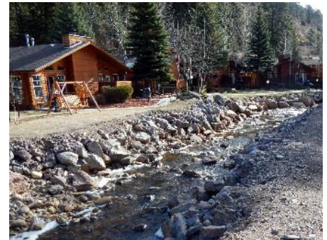
Picture 1: A constrained river between two rip-rapped banks
