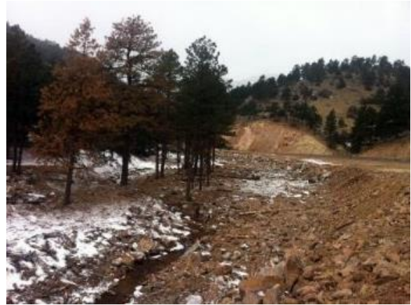
Picture 8: Meandering multi-stage channel (with water in the low-flow channel) on the Little Thompson River near Pinewood Springs, Colorado
