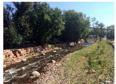
Picture 2: An accommodated river with protection adjacent to homes, riparian vegetation, and space for flows to expand
