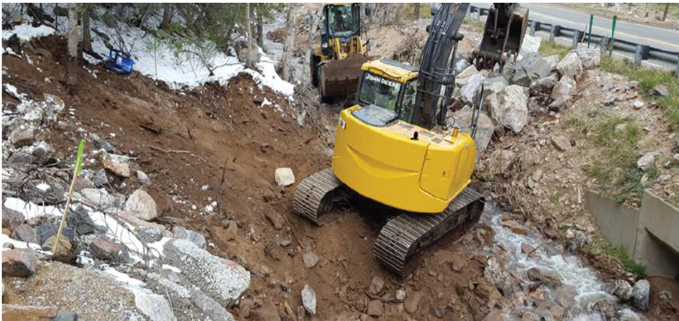
Above: Crews install bank protection to protect critical highway infrastructure. Below: Volunteers harvest willows for revegetation.
