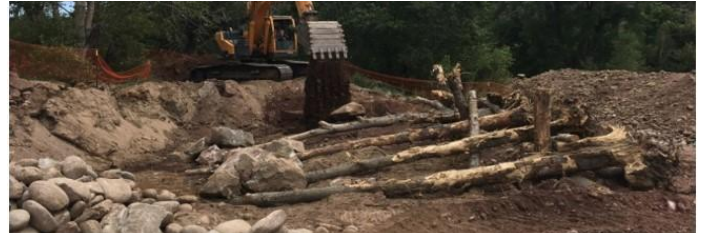
Installation of large woody structures within the project area.
