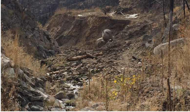
Upstream end of the project reach showing extensive erosion and evidence of debris flows and sediment deposition.
