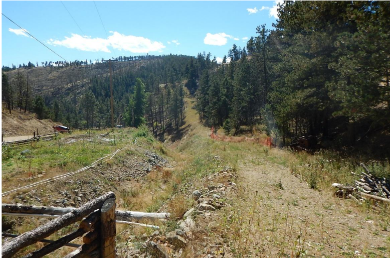
Looking downstream at the lower portion of the project. Note steep banks, lack of floodplain, and extensive deposition.
