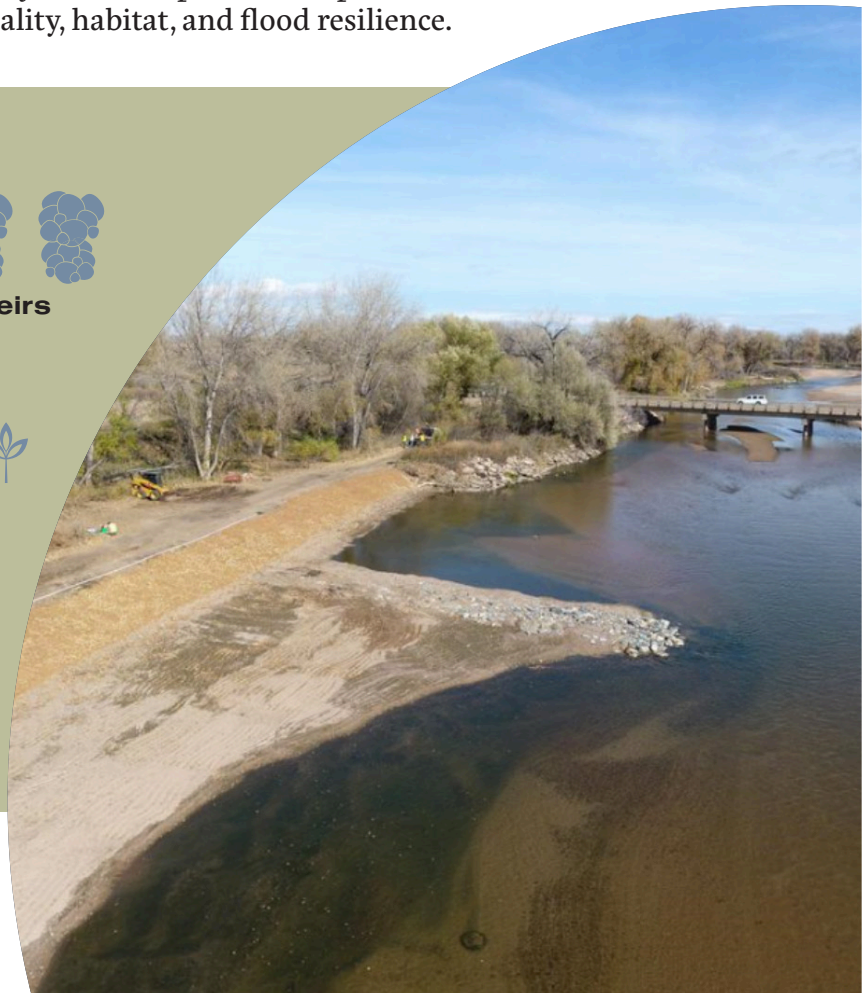
Post-construction aerial view of Weir 1 and the SH 60 bridge looking east.
