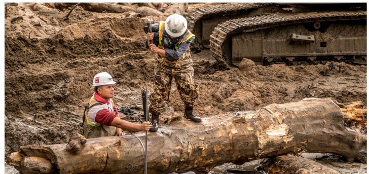
Installing woody material to provide aquatic habitat.
