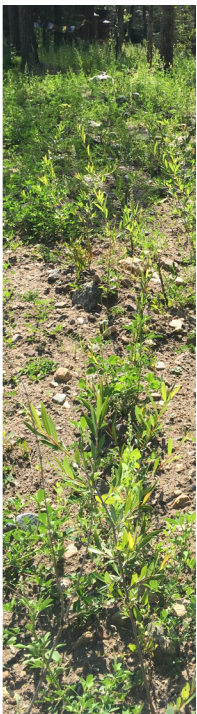
Left: Willow toe, a bioengineering treatment, taking root along Upper Fourmile Creek. Top: One of two new diversion structures installed during construction of the Wall Street project. Bottom: Work to increase channel capacity.
