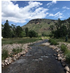
North Saint Vrain Creek at Apple Valley after construction (July 2018).
