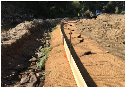
Left and Bottom: Construction of soil-wrapped lifts, including live willow installation.
