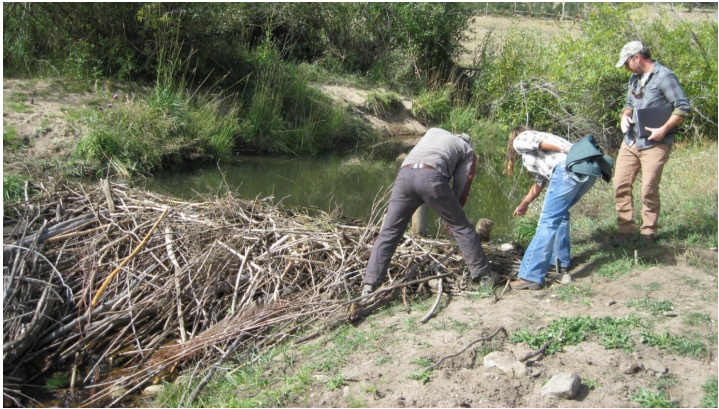
Installation of a beaver dam analogue.
