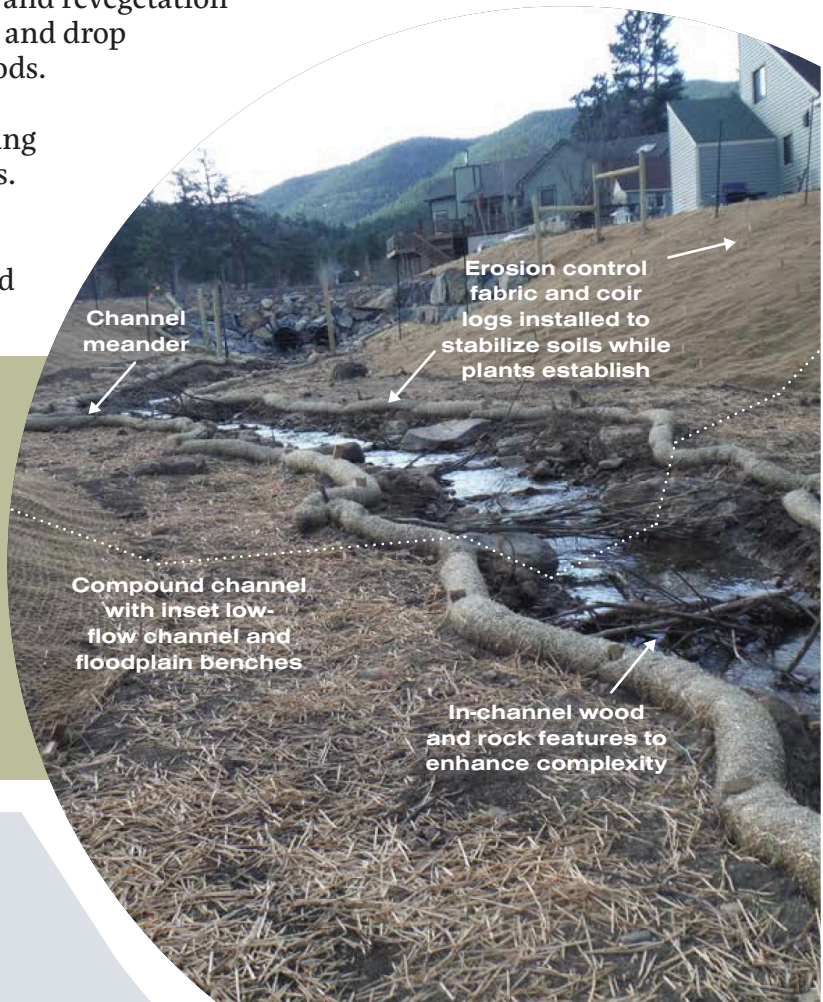
Reach 5 looking upstream just after construction, featuring a compound channel with improved floodplain access, meanders, in-channel complexity, and soil stabilization through coir logs and erosion control fabric.
